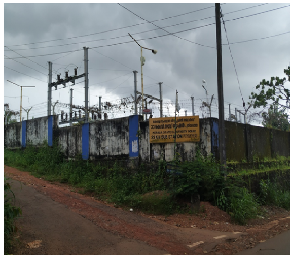
Puthiyatheru 33 kV Substation (Podikkundu- Kottali Road)
